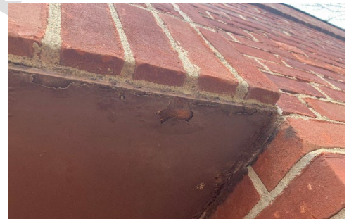
19: Close-Up View of Underside of an Exterior Lintel
