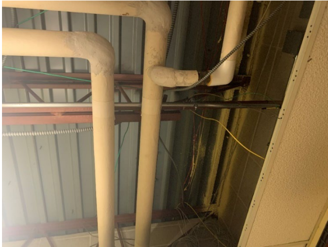
10: Underside of Typical Classroom Roof Framing in 1978 Wing
