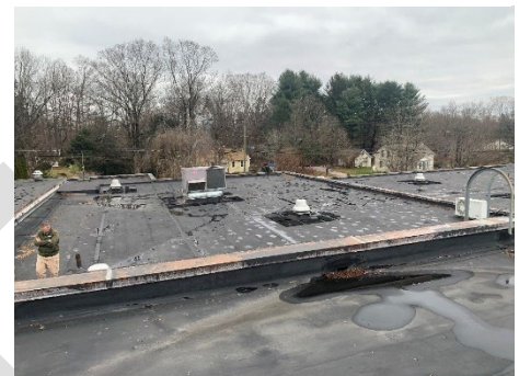
5: Partial View of Roof (Looking East)
