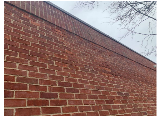
5: Partial Exterior Elevation View of Brick Masonry Veneer
