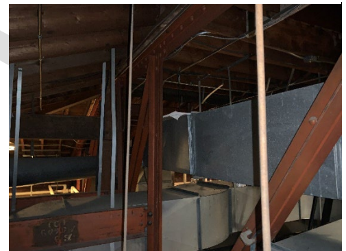
16: Partial View - Sloped Roof / Attic Framing
