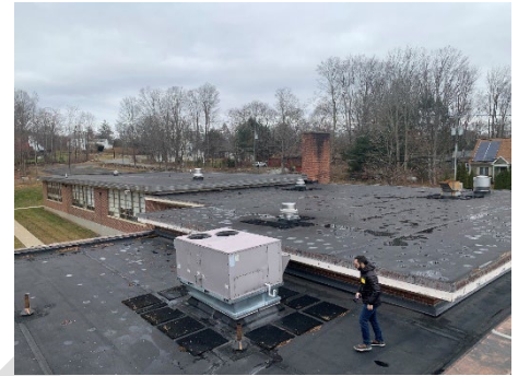
4: Partial View of Roof (Looking Northeast)
