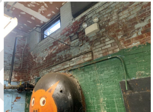
211: Interior Face of Interior Boiler Room Exterior Wall
