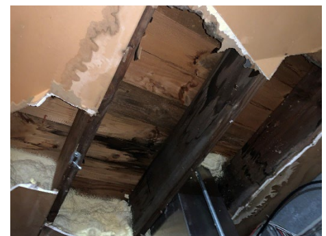
9: Underside of Wood Roof Framing in 1952 Upper Wing
