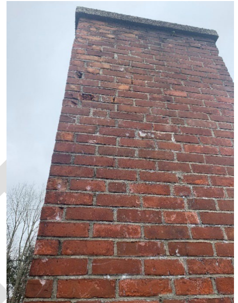
7: Close-Up of Western Chimney Elevation Above Roof (Looking East)
