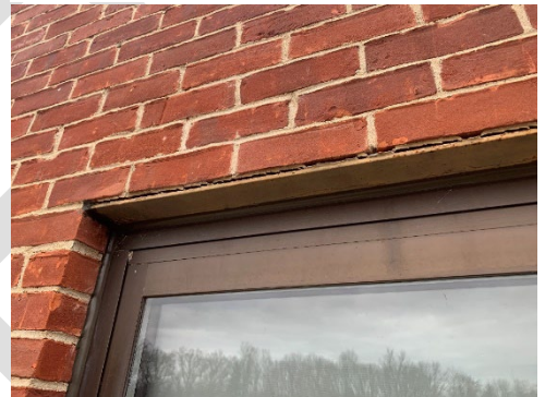
18: Close-Up of a Lintel Over an Exterior Window
