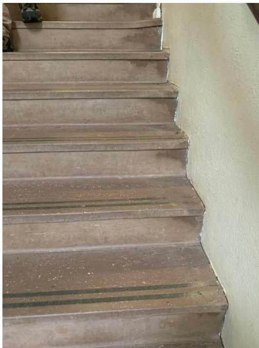
14: Partial View of Existing Interior Stair by Southern Entrance
