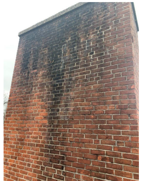
6: Close-Up of Southern Chimney Elevation Roof (Looking North)
