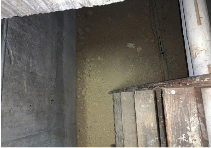
13: View of Tunnel Access Opening / Pit Floor
