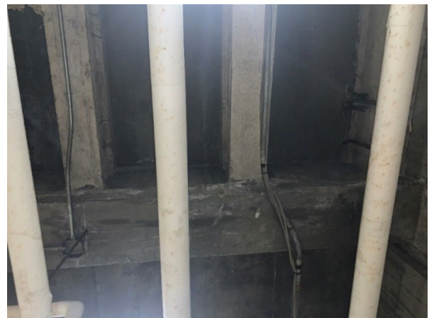
124: Underside of Concrete Floor Framing Above Mechanical Room
