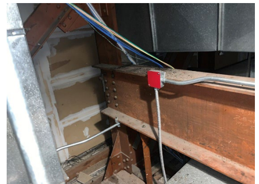
17: Close -Up View Attic Truss Framing Connection
