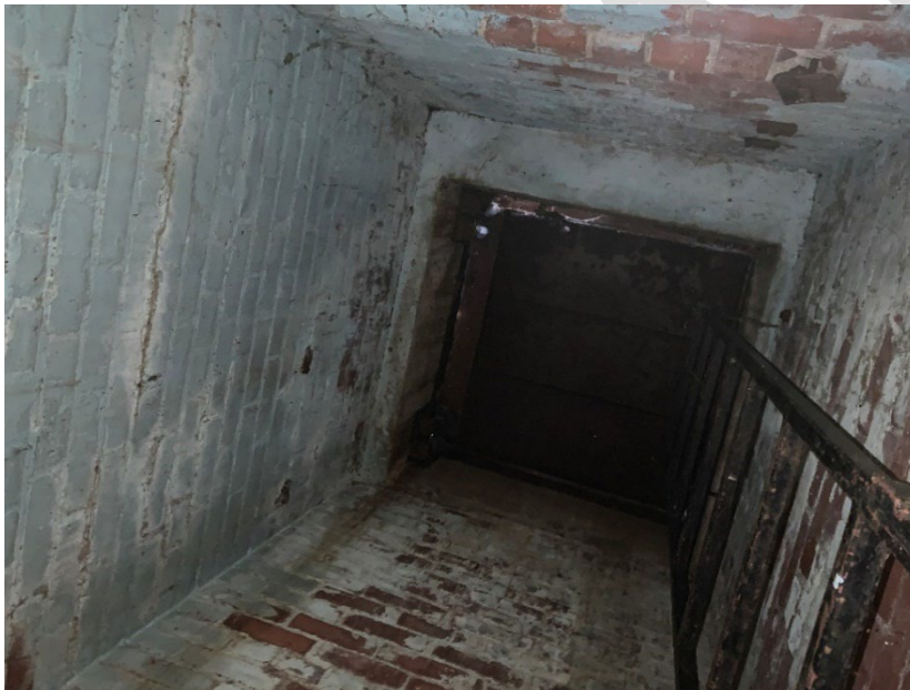
10: Mechanical Room Masonry Shaft (looking up)
