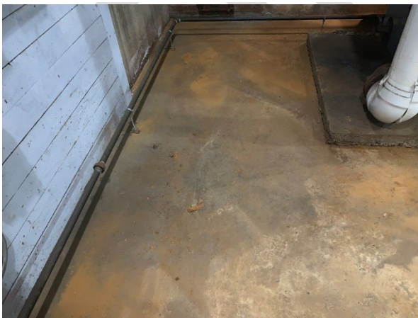
15: Partial View of Slab-On-Grade in Mechanical Room
