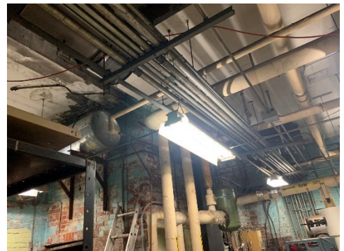
8: Underside of Floor Framing Above Boiler Room
