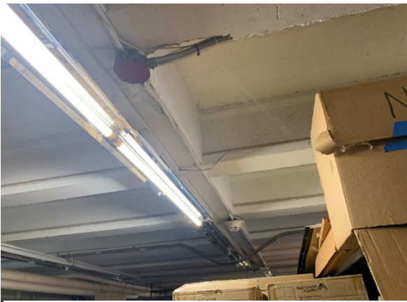
12: Underside of Concrete Floor Framing Above Storage Area
